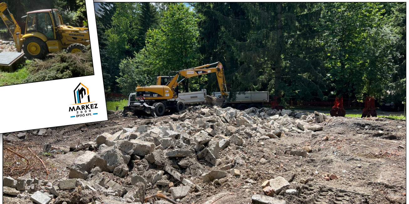
Demolition of a Military Resort (Anna-völgy)
