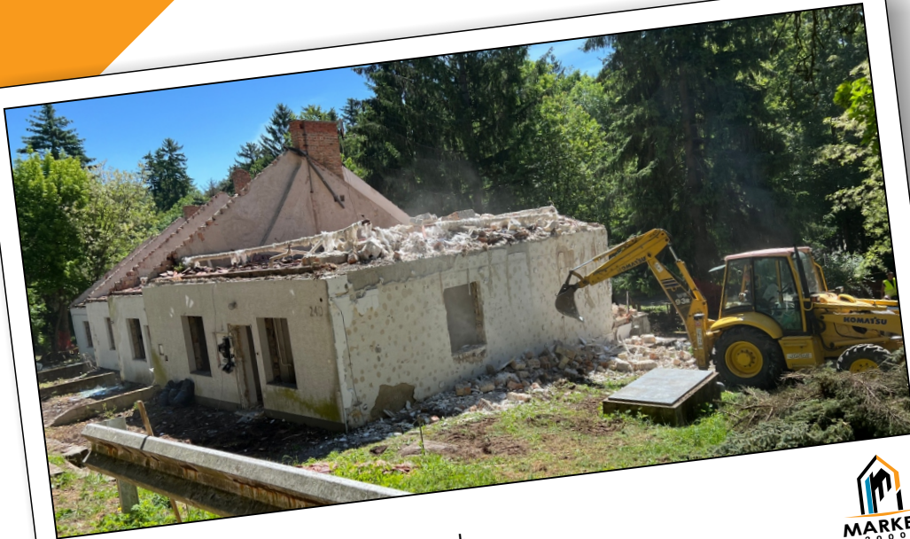
Demolition of a Military Resort (Anna-völgy)
